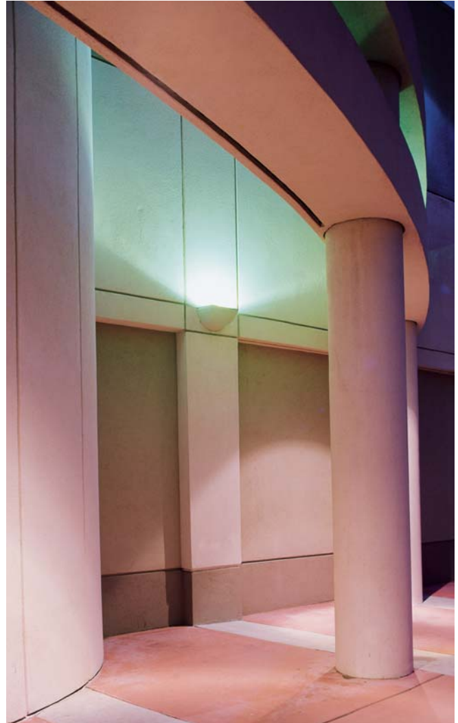
Tucking a sconce into discrete locations adds a dramatic effect, improving security and making the building come alive at night.
