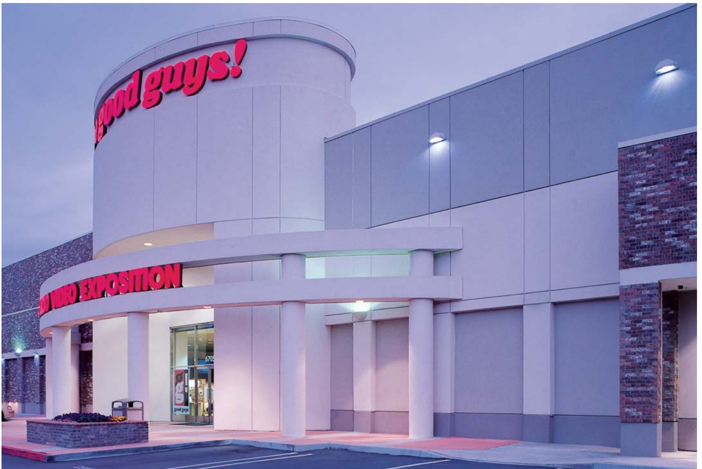
Combining standard downlight sconces with inverted sconces allows for the right amount of light in all the right places around the building.
